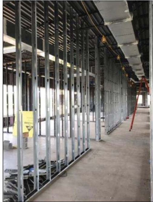
Main Building (Interior Metal Studs)
