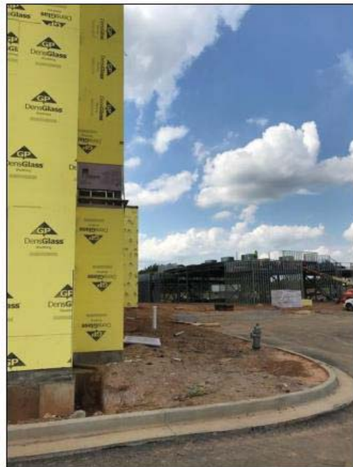
Auditorium (View Northwest)
