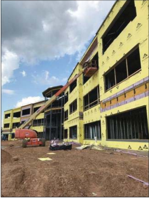
Main Building (View Northwest)
