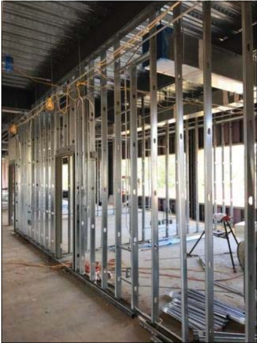
Main Building (Interior Metal Studs)
