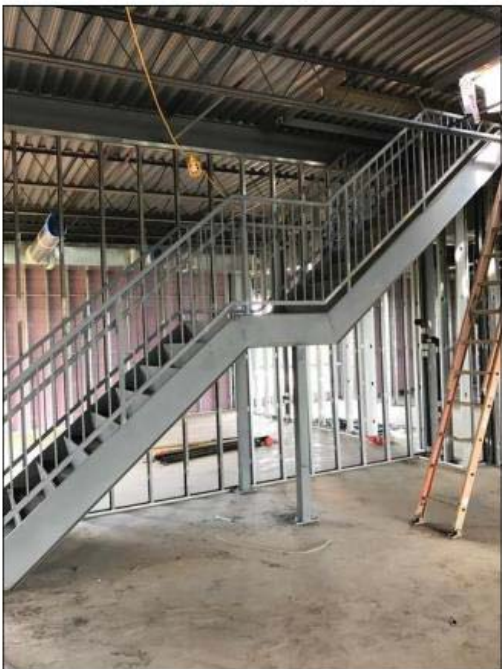
Main Building (Roof Access)
