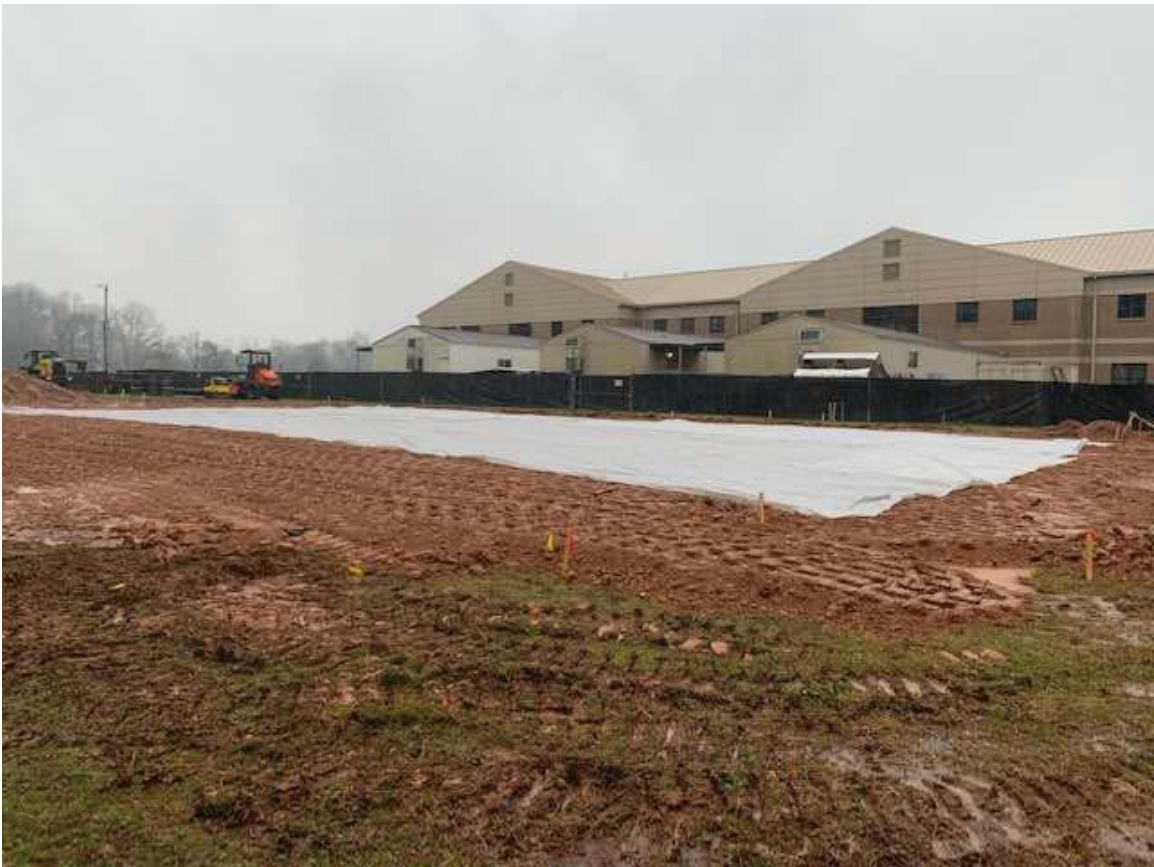
Site Grading – Pad Prep
