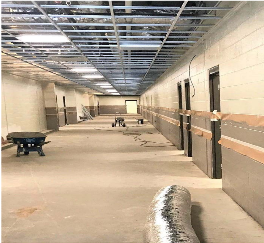
1 st Floor Hallway
